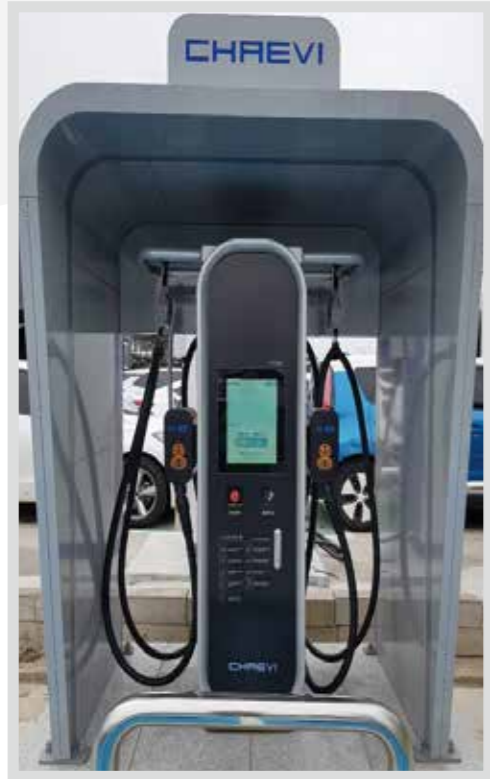
15" Panel pc installation in Jeju Island
