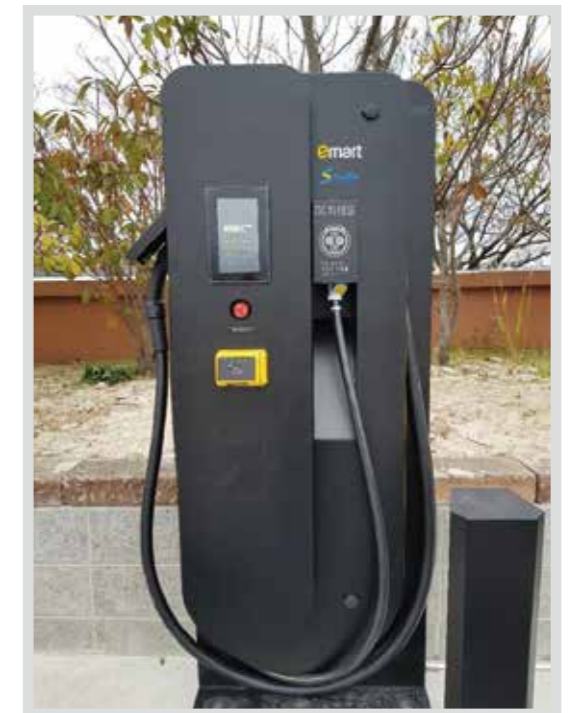
8" Panel pc installation in Jeju Island
