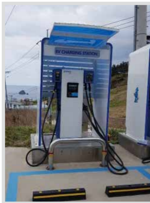
8" & 12.1" Panel pc installation in Ulleungdo Island
