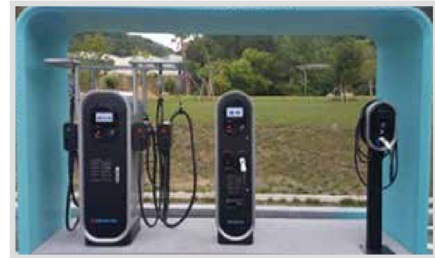
8" Panel pc installation in Jeju Island
